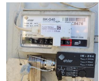
FM432g-n on a gas meter
